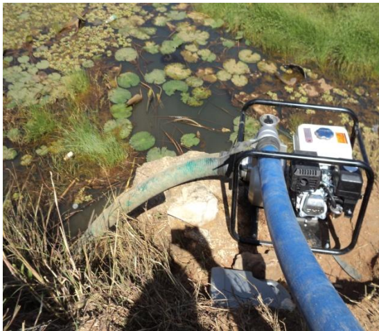
Fig 3. Pump machine in the excavated pit
